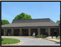
Tucker Nursing Care Center - Roddey (General Nursing Home) - a 185-bed skilled nursing care facility located in Columbia.
